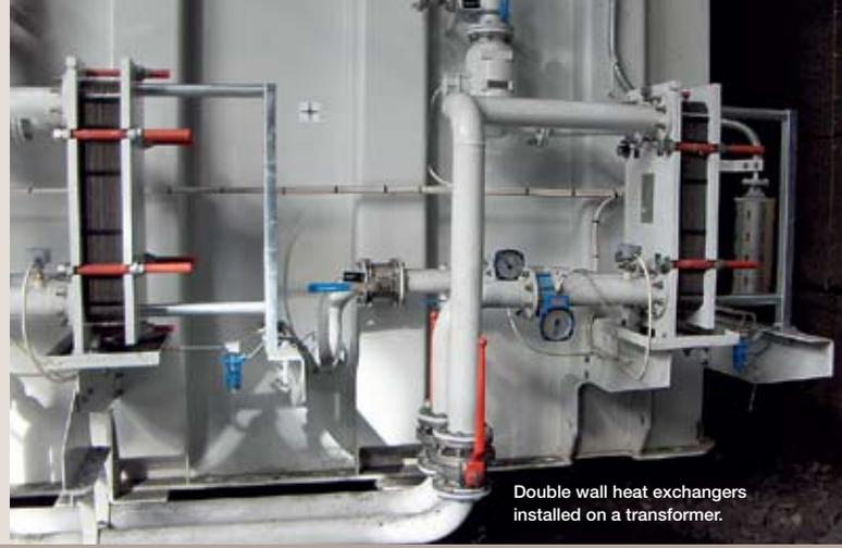
Double wall heat exchangers installed on a transformer.
